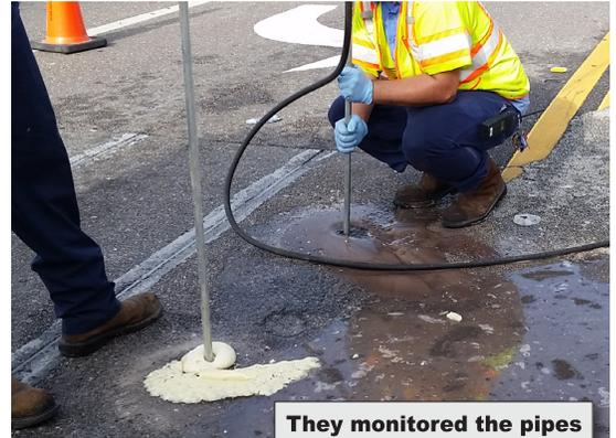
They monitored the pipes while injecting material at a rate of 2 gallons per vertical foot through the open manhole to identify additional leaks that had been missed during the first point repair.
