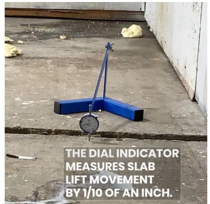
THE DIAL INDICATOR MEASURES SLAB LIFT MOVEMENT BY 1/10 OF AN INCH.
